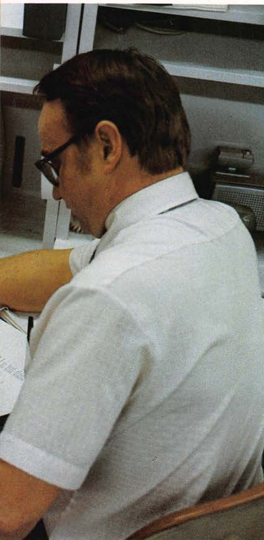
WE Installers Frank Regan and Bill Sumski at the maintenance console of Cedar Knolls 5ESS* switching center.
