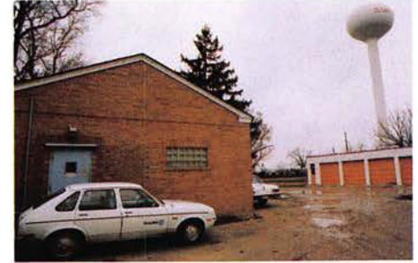
Illinois Bell's step-by-step office was located in this rented building hidden behind the village general store.
