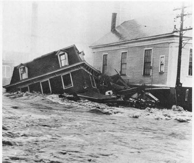
Floods again. This time, the scene is New England, where a hurricane swept central offices away in towns like Ware, Mass., above, and halted service for some 515,000 telephones. Repair crews from as far away as Southwestern Bell territory were mobilized to deal with the emergency and get things back to normal. The year was 1938.
