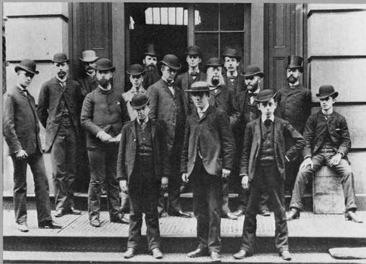
Staff of the New York branch the year we entered the Bell System. We rented the building from Western Union. American Stock Exchange and NYU Business School now occupy the block.
