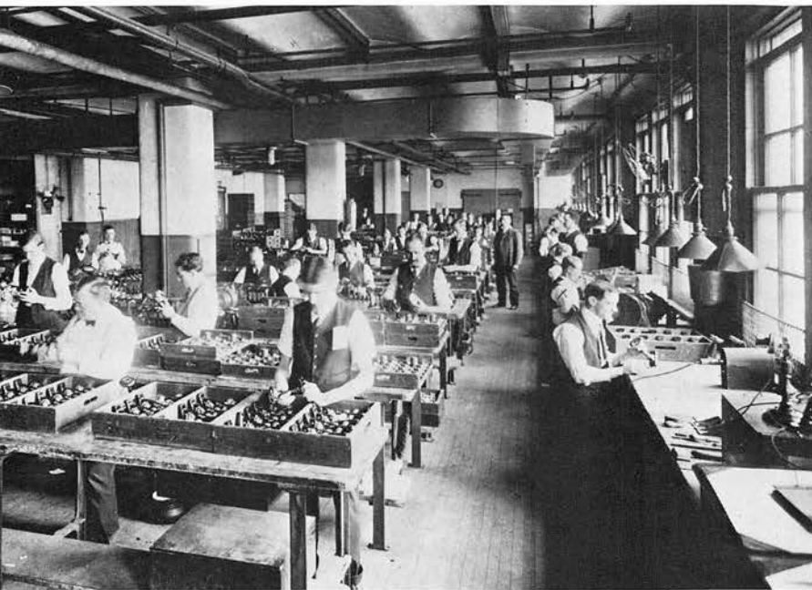
1905 —The term “mass production” hadn’t taken on meaning yet. These workers are assembling telephone transmitters. The workers in the 1895 photo (left) would have experienced no future shock in this shop.
