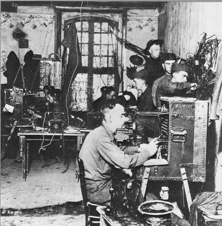
In France during World War I, vital messages were switched over this WE "Camp" switchboard, one of many special products we made for the armed services.
