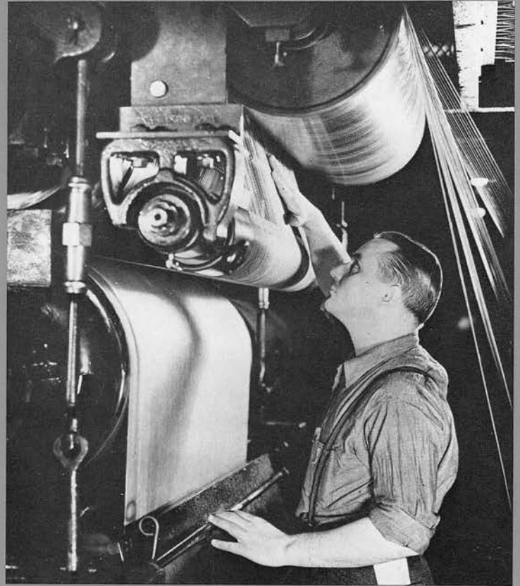
One of the major production advances during the 20s was the introduction of pulp insulation on cable. This photo is from the then brand new Kearny Works.
