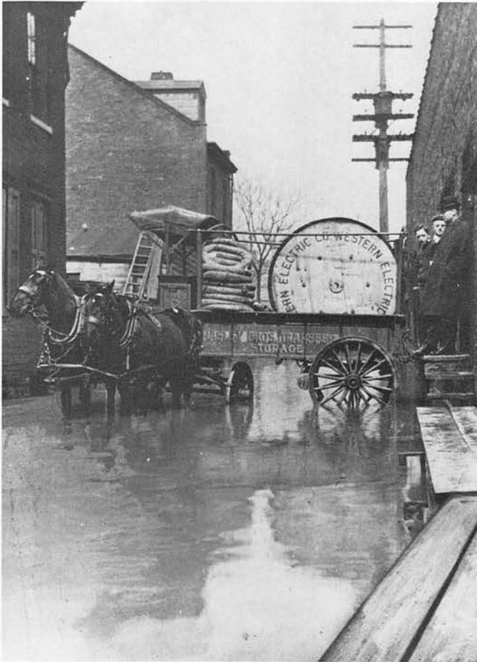
The year was 1913, and a lot of Pennsylvania was under water. This WE cable being loaded in Pittsburgh helped restore communications. So did the two-horsepower wagon.
