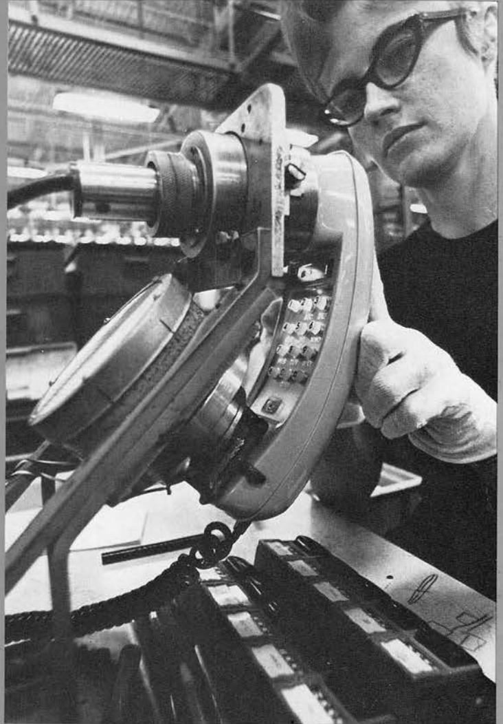
Above—The Trimline® telephone and Touch-Tone® calling, two of the major innovations in station equipment during the 1960s are combined in this photo of the final test operation at Indianapolis.
