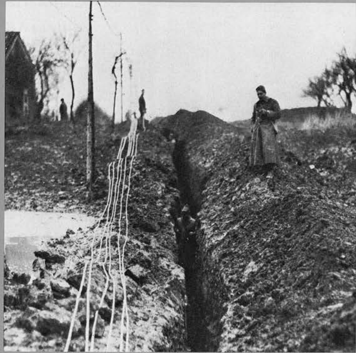
Trenches and World War I go together. This one near Ausauville, France, was for telephone cable. Like many during the war it was dug under continuous German battery gun fire. The date on this is 1918.
