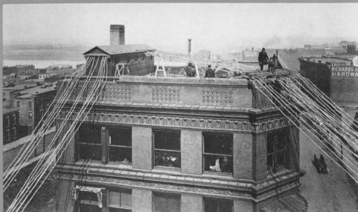
This was the telephone exchange in Kansas City, Mo. in 1895, when WE installers were putting in a new exchange. All wires still came in over the rooftops.
