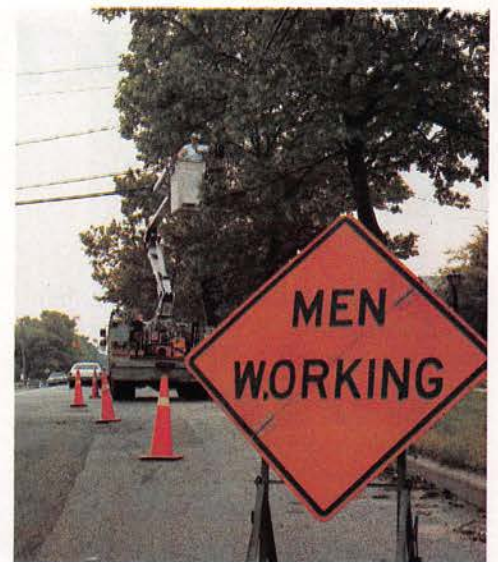
Sometimes, you need a cherry picker to work on the loop.
