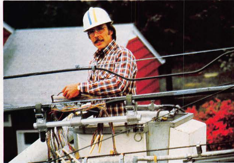
splicing cable between utility poles
