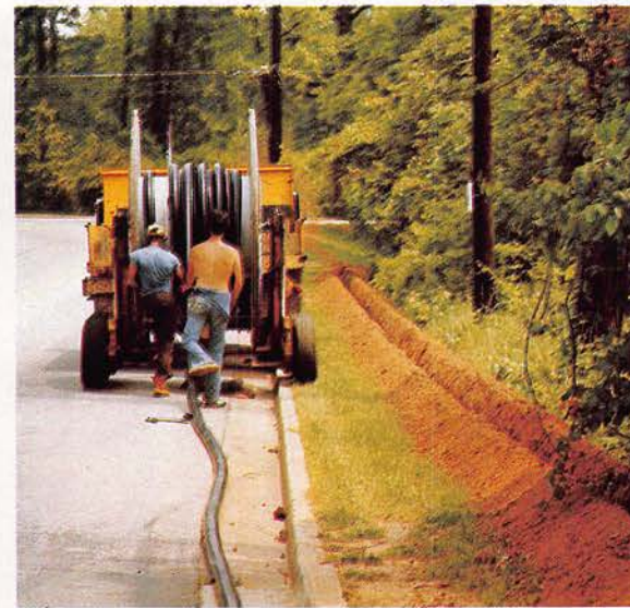
Unreeing some new cable in a suburban Atlanta community.
