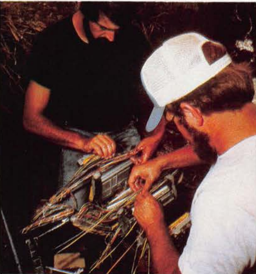
These 710 connectors simplify the splicing of aerial cables.
