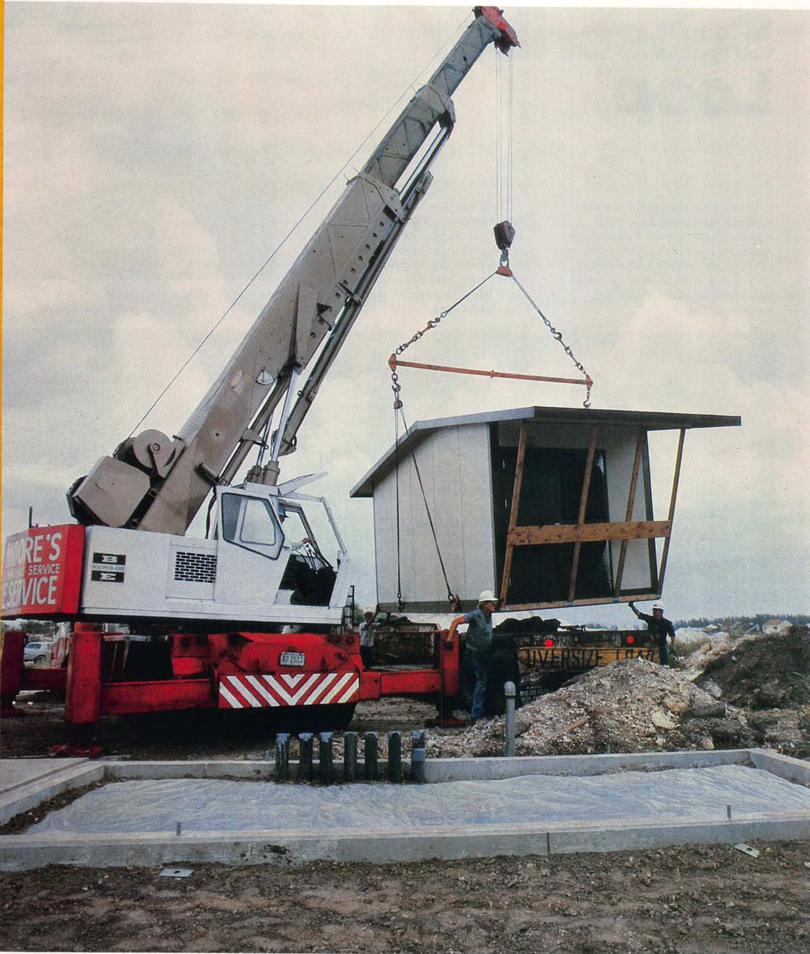
WE engineers from Atlanta oversee placement of a SLIC-96 maxibut in a new housing development in Miami.
