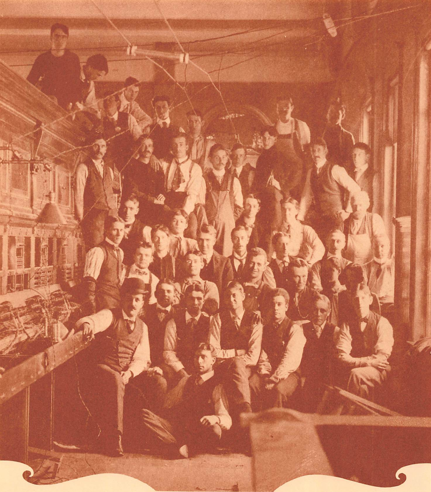
Switchboard installation in Oregon, 1900.
